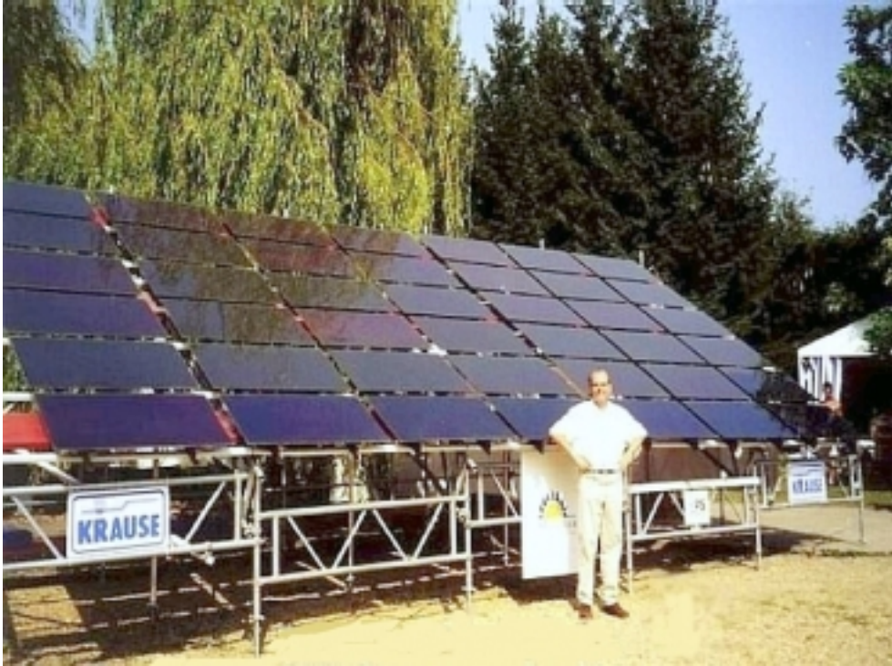
Solar System 1500W with 64 pcs. of solar modules (Obuda Island)
